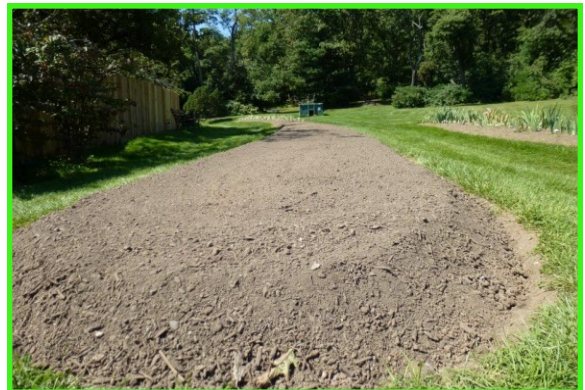
One of the iris beds during renovation
